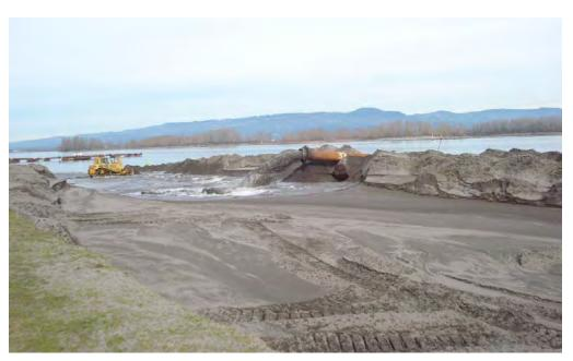
Figure 11: Active shoreline placement at Sand Island (looking downstream)
