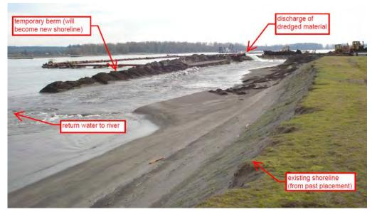
Figure 10: Active shoreline placement at Sand Island (looking upstream)
