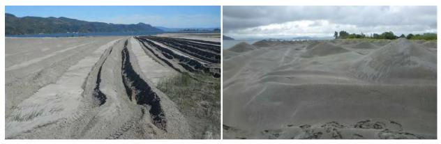
Figure 3: Trenches on Rice Island (left) and mounding on Miller Sands Island (right)
