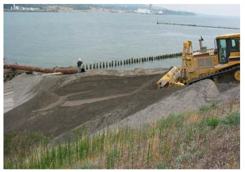
Figure 6: Grading slope for incoming dredged material pipe
