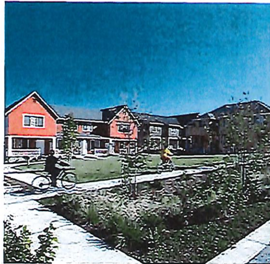
Homes front onto common greens.
