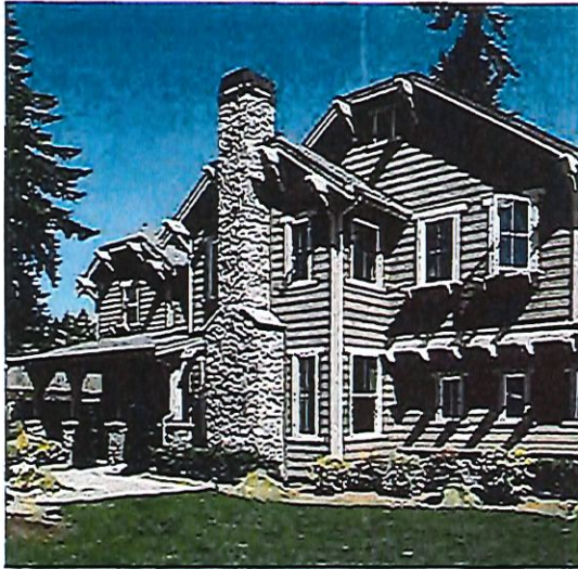
The Woodlands district encourages architecture that has its forms and materials drawn from mountain architecture.
