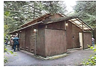
PHOTO OF EXISTING
