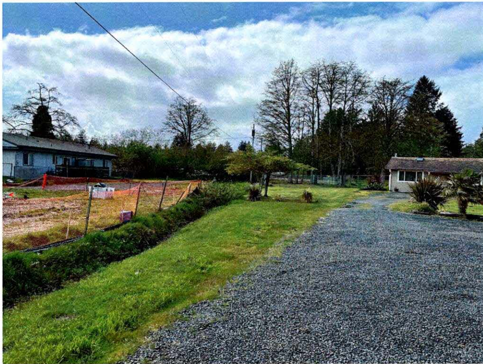
Location of 7th street half street improvement.
