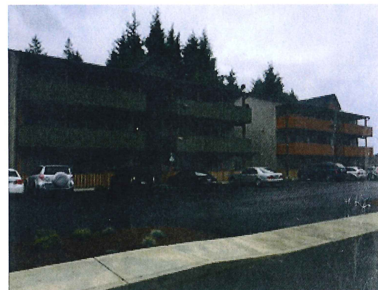
Completed Apartment Building - Similar Design
