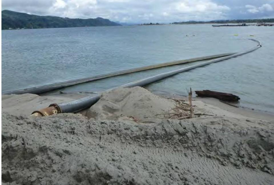
Figure 8: Outfall pipes returning water back to river after dredged material has settled out, Rice Island
