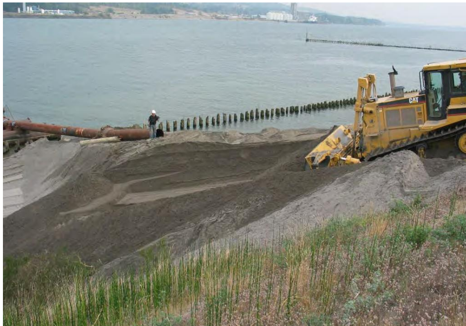
Figure 6: Grading slope for incoming dredged material pipe
