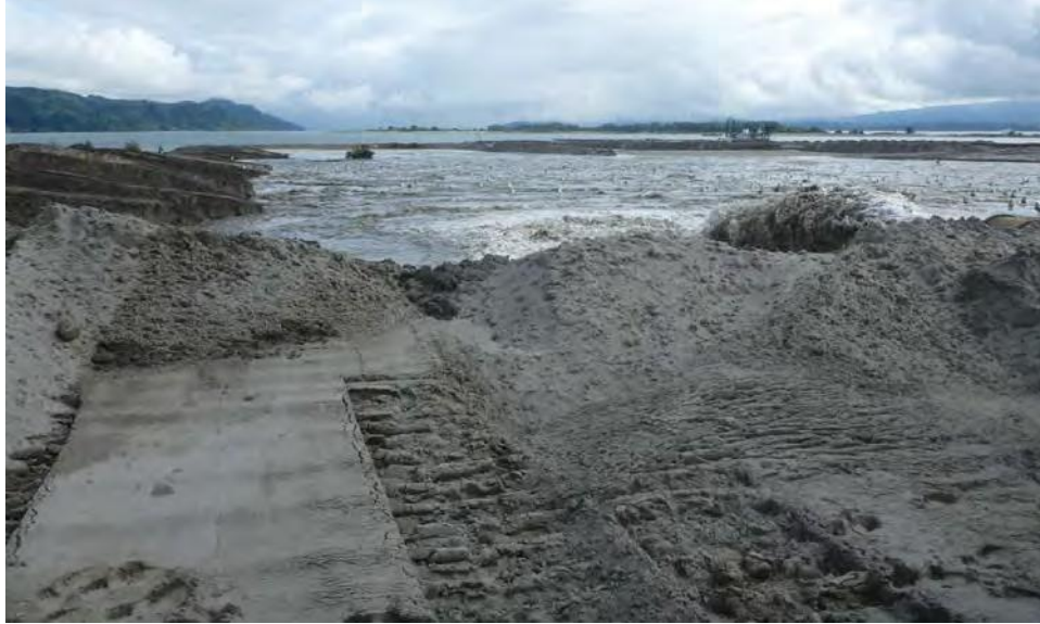
Figure 13: Active discharge of sand and water dredged material slurry at Rice Island Upland Site
