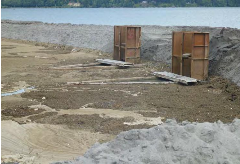
Figure 7: Weir and berm structure, in operation on Rice Island
