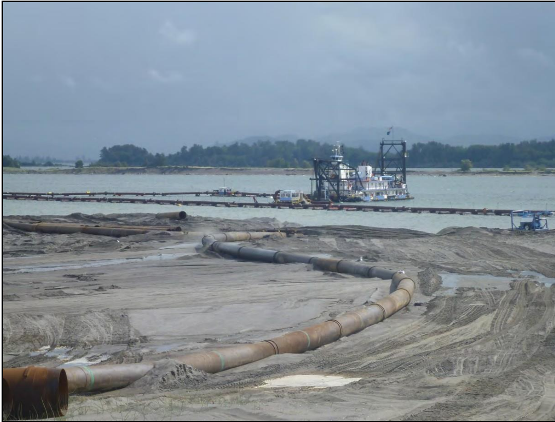
Upland placement of dredged materials on Rice Island, September 2013
