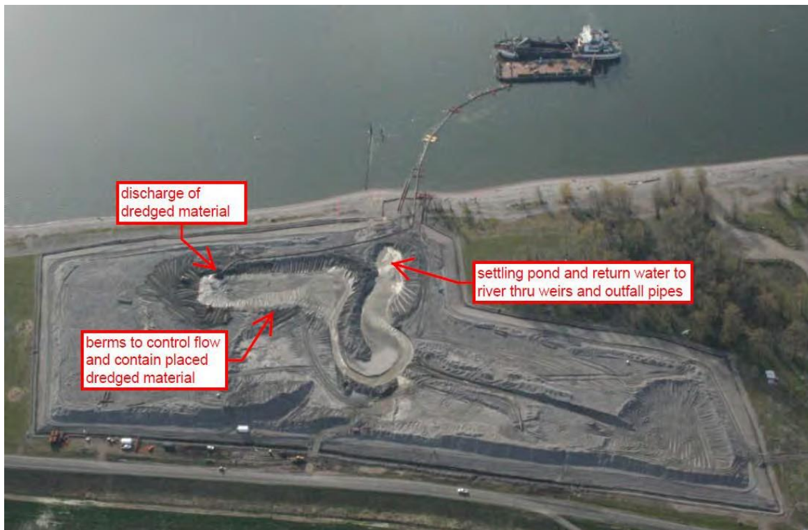
Figure 12: Active dredged material placement at Martin Bar Upland Site
