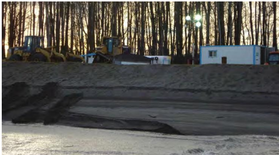
Figure 9: Staging equipment on top of the bank at Sand Island Shoreline Placement Site
