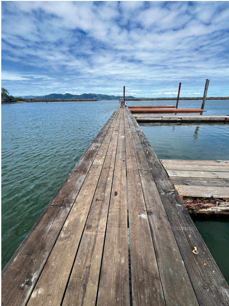
SECTION OF D DOCK THAT HAS BEEN REBUILT
